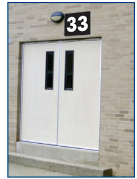
Exterior door with number on building
